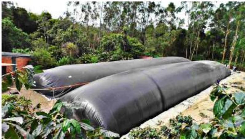
Figura ~~3637~~. Biodigestor Taiwan. Fuente: (Shemi,2015)
