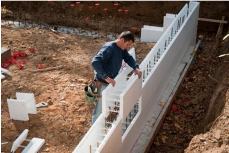
Fuente: (Insulating Concrete Forms Foundation, 2016)
